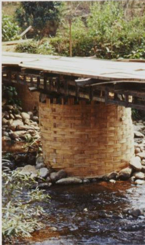
A bridge supported by stones wrapped in a bamboo basket (suburb of Vientiane, Laos).
